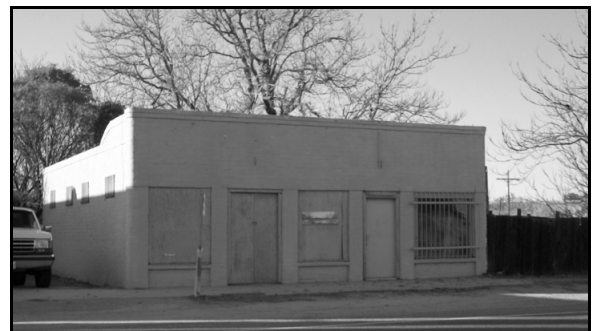
Vacant building on Friant Road
